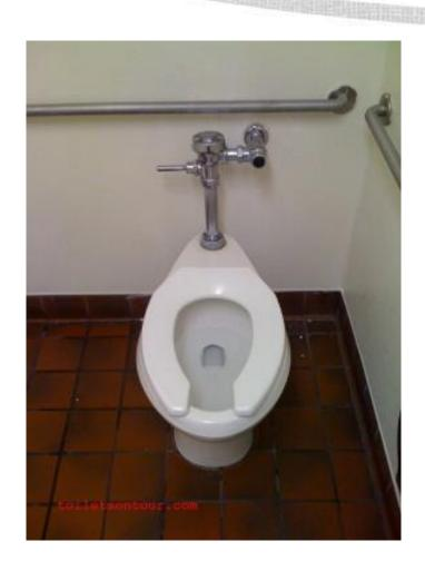
Grab bar placement in relation to water closet flush valves
