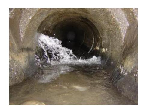
Sanitary and storm sewer piping is shown with a slope less than the minimum allowed by code
