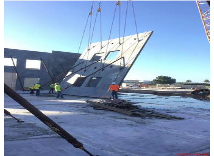
Erecting of Tilt Panels
