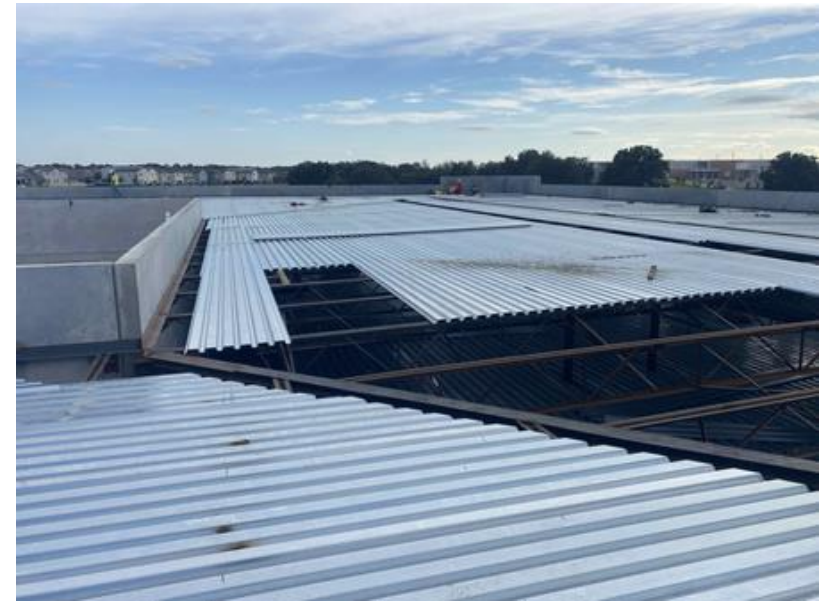
Roof Metal Decking
