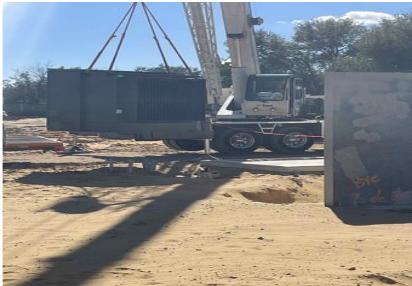
Main Electrical Transformer set and Energized
