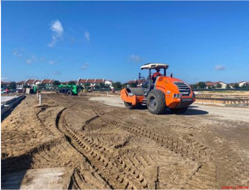
Compacting Access Roads and Building Pad
