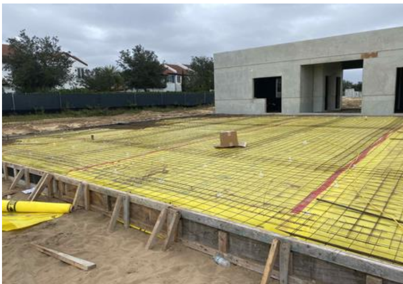
Foundation Slab for PE Building getting Formed
