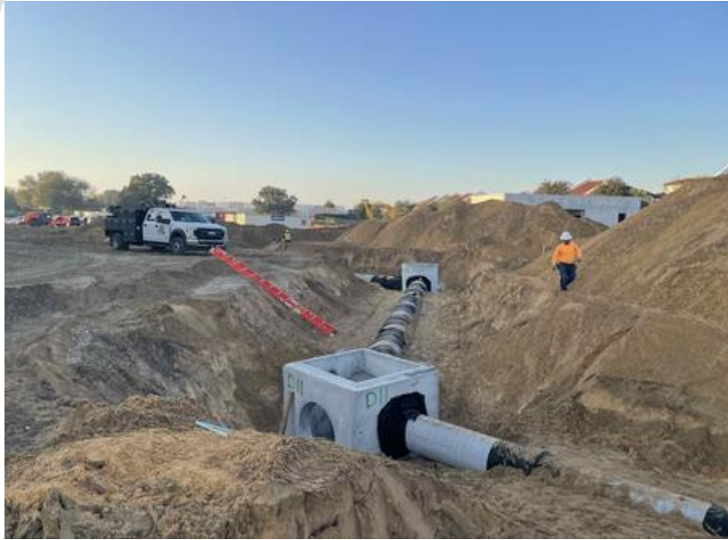
Installation of Civil (Storm) Underground Ongoing
