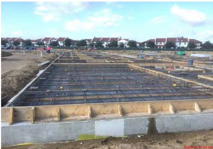
Tilt Panel Forming and Steel Reinforcement
