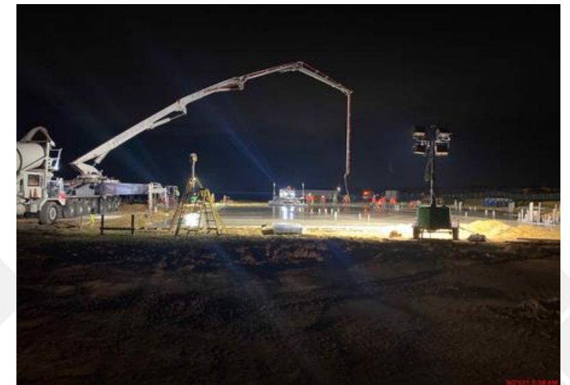
Early Morning Pour for Panels and Casting Slabs
