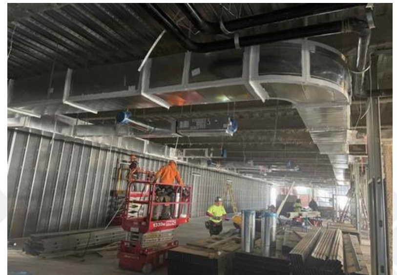
Above Ceiling Mechanical Duct being installed
