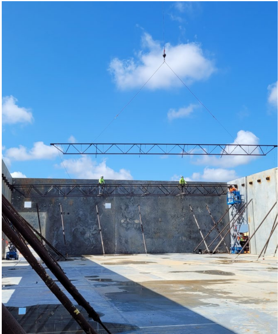
Above is placement of steel joists
