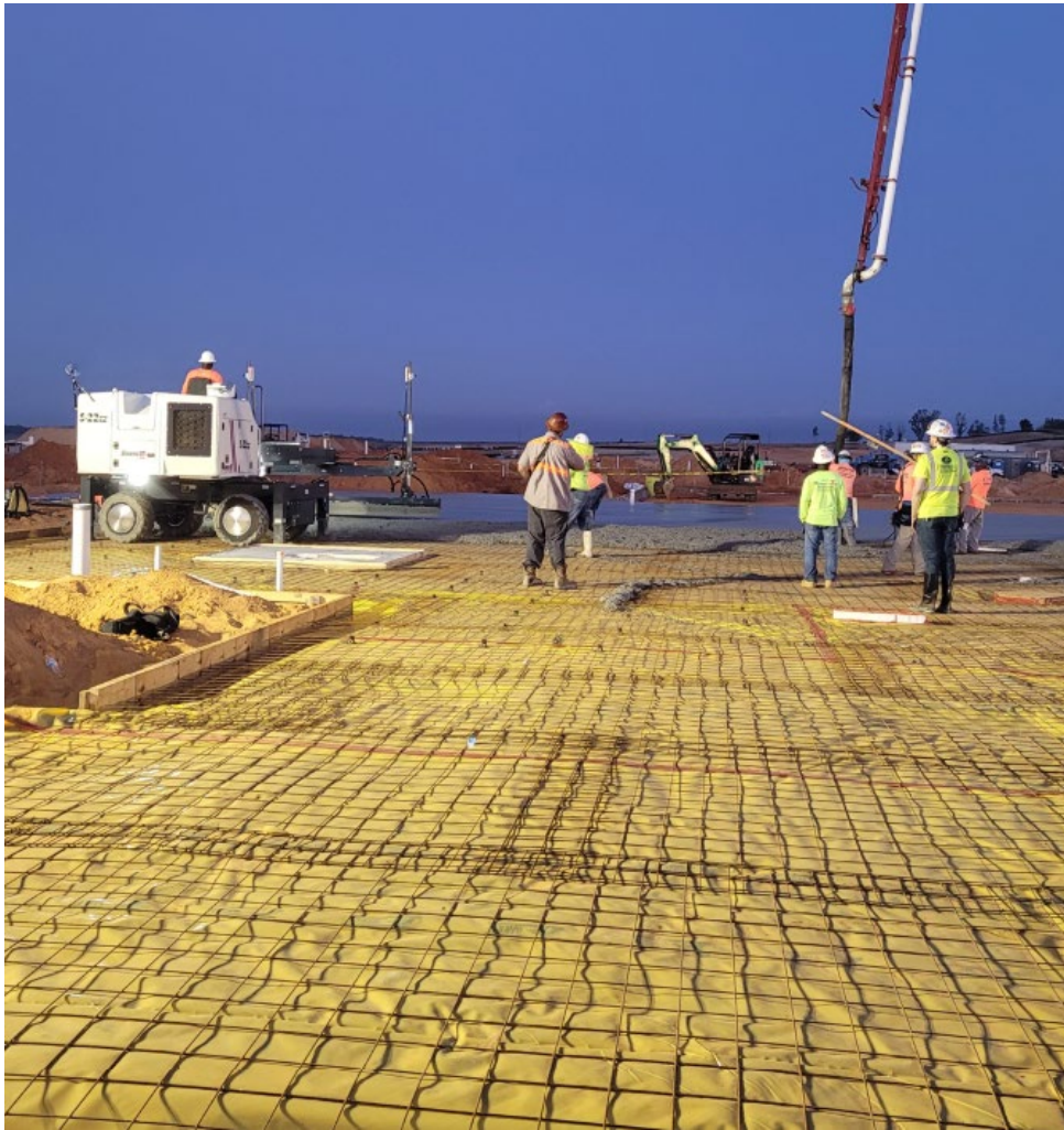
April - above is Slab on Grade pour of Building 4 looking west
