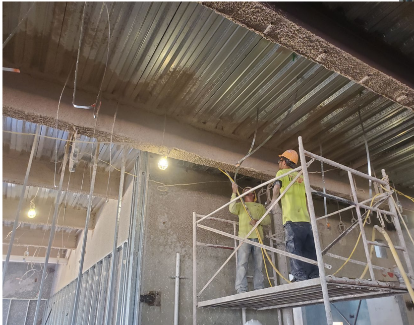
Below is firespray placement on Building 5 steel beams
