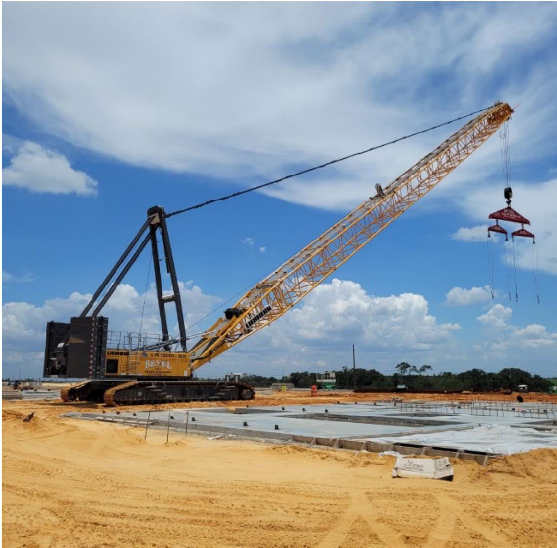
Above is prep of crane for tilt panel erection
