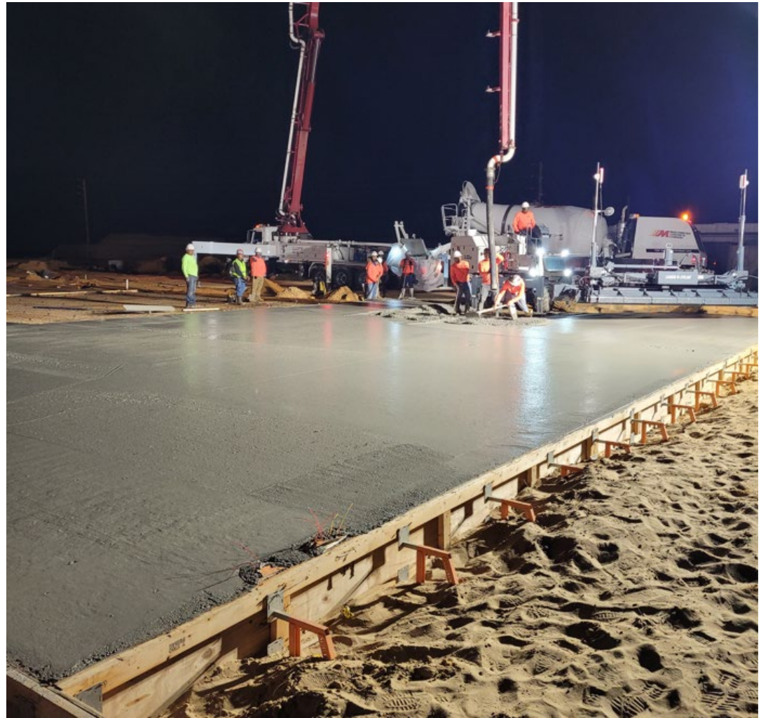
May - above is Slab on Grade pour of Building 2 looking west
