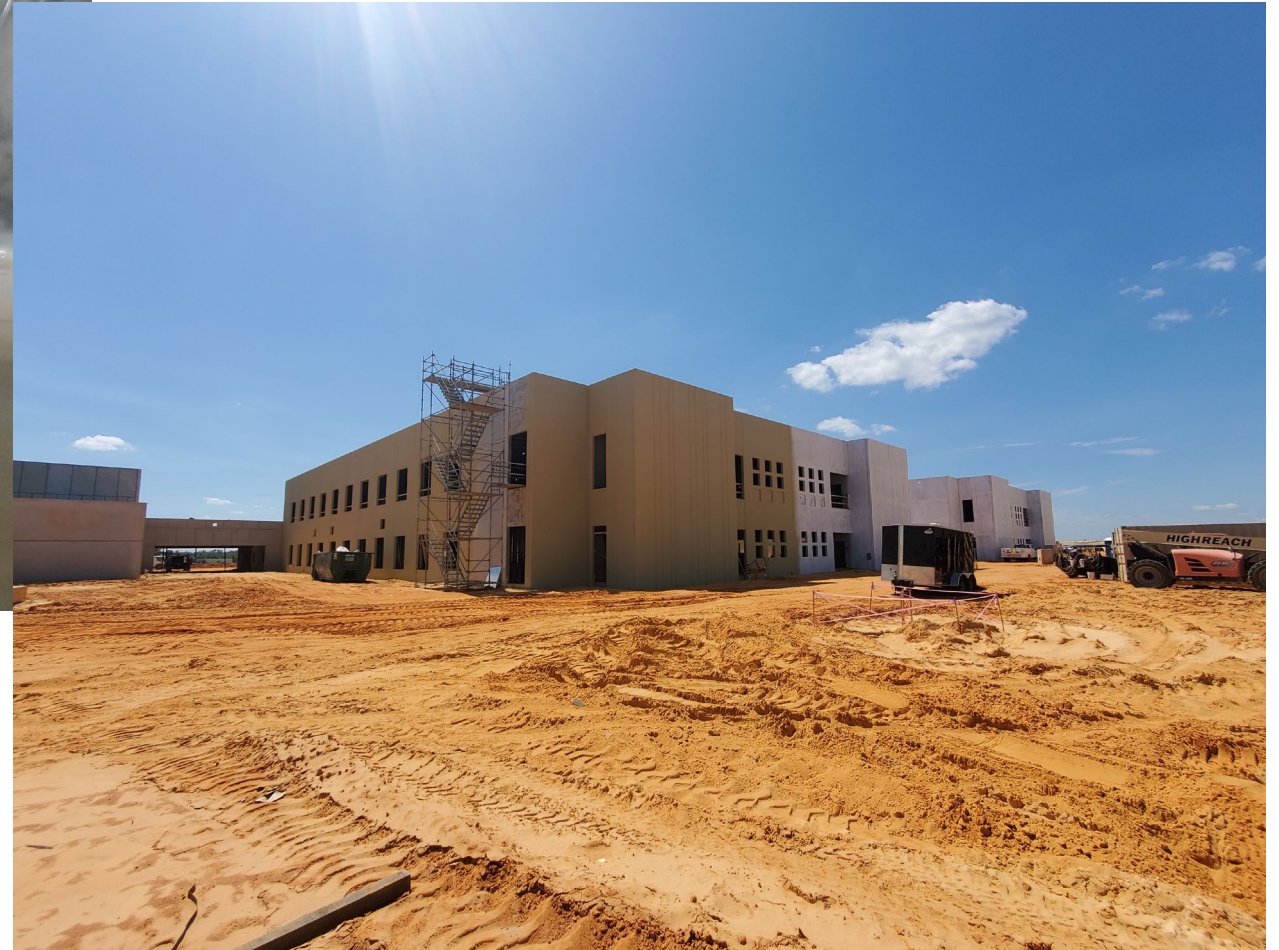
Below is prime paint and texture coating on Building 5 tilt panels from NE looking SW
