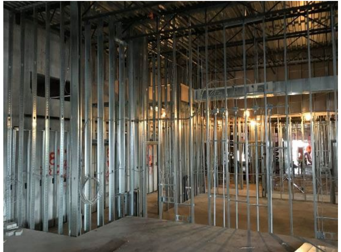
Interior Classroom Framing
