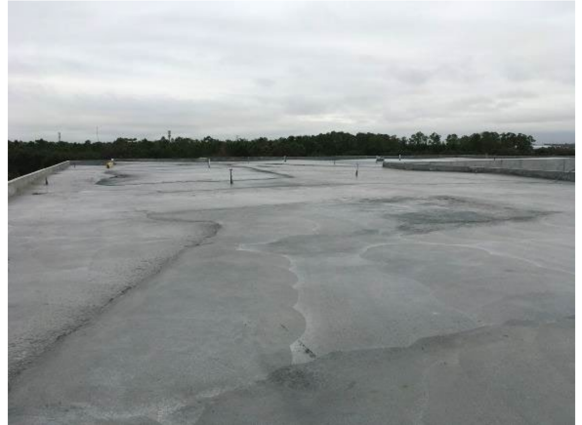
Lightweight Insulating Concrete
