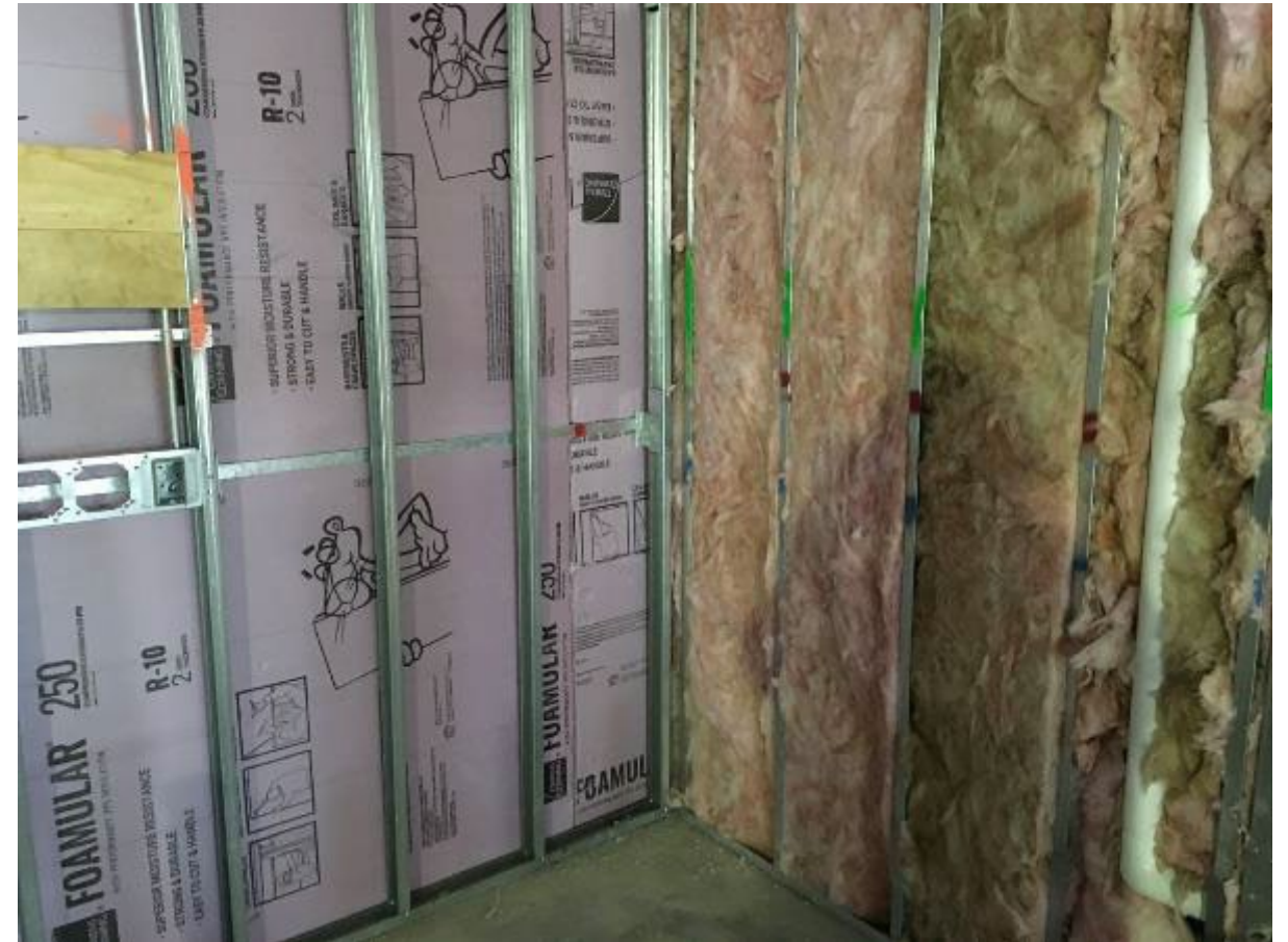
Interior Wall Insulation
