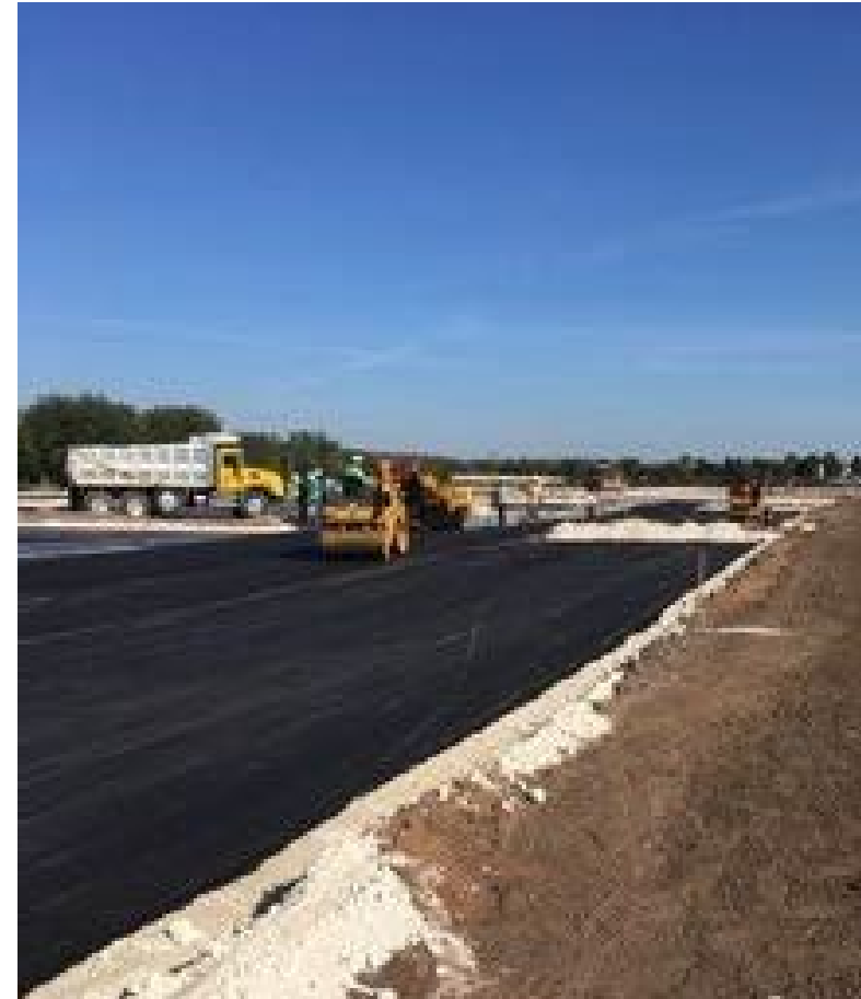
Asphalt paving for Parent Parking
