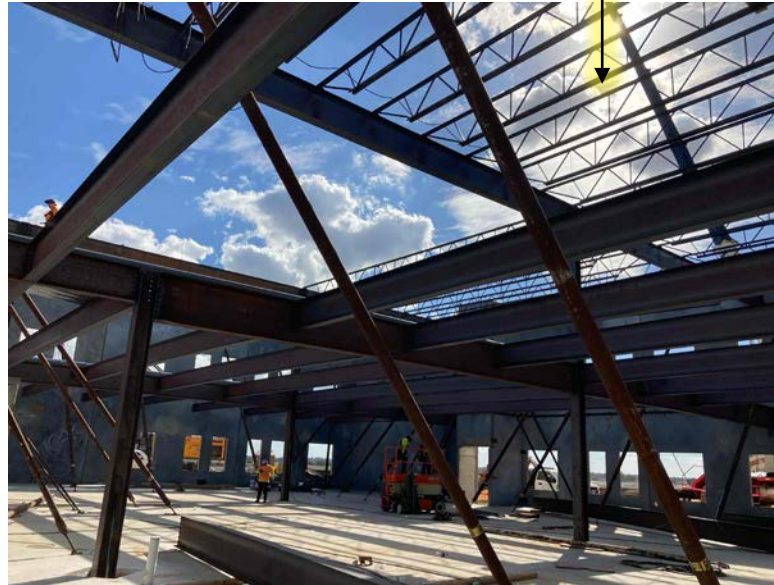
Erection, bolting and welding of structural steel beams, columns and joists.
