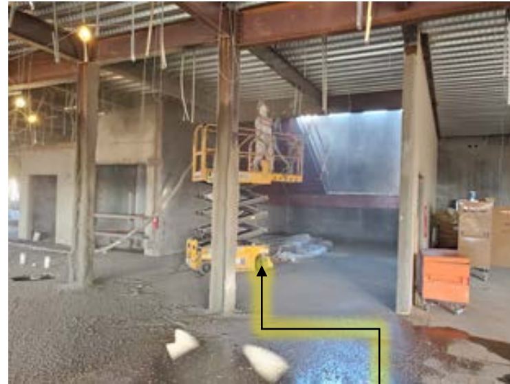
Fireproofing of columns, beams and joists
