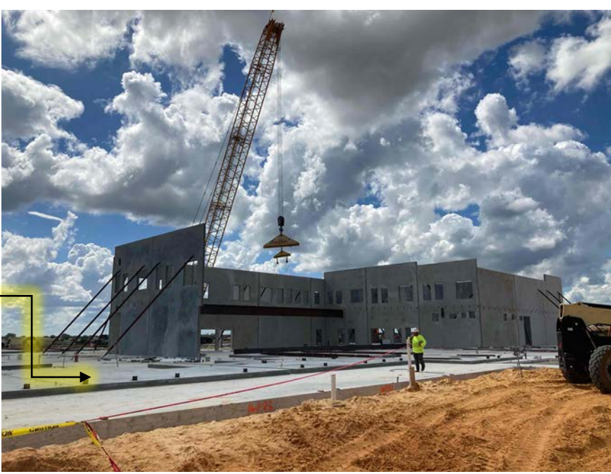
Tilt panels erection and bracing
