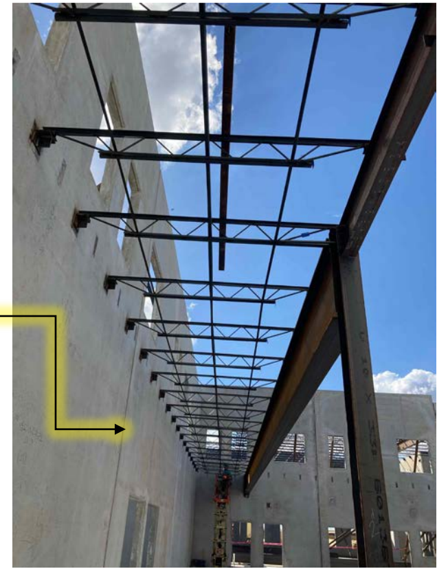
Erection, bolting and welding of structural steel beams, columns and joists.
