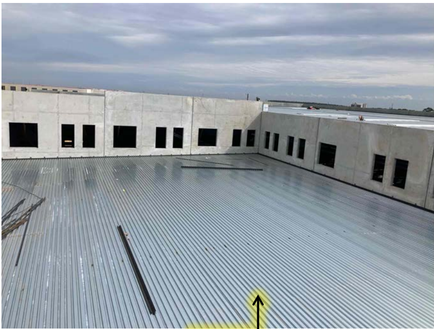
Roof decking install complete at Low & High Roofs
