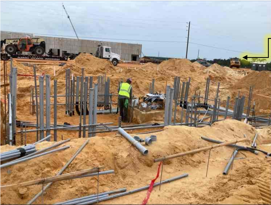
August: MEP rough-in and Slab on Grade prep
