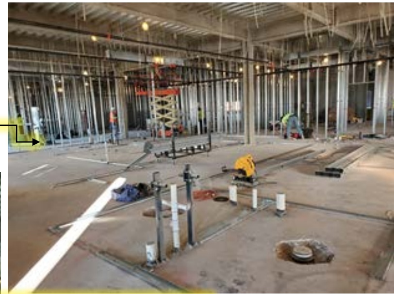
Metal framing and MEP wall rough-in in progress on 1 st floor
